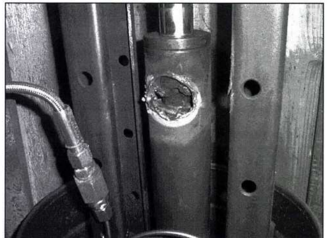
Homemade booster that combusted while boosting 50/50. There was a threaded port and hose where the hole is now.
